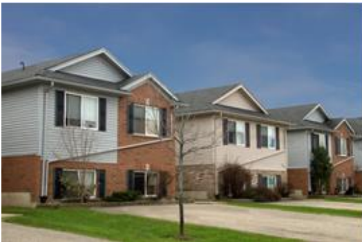
Village Road Built – 2004
