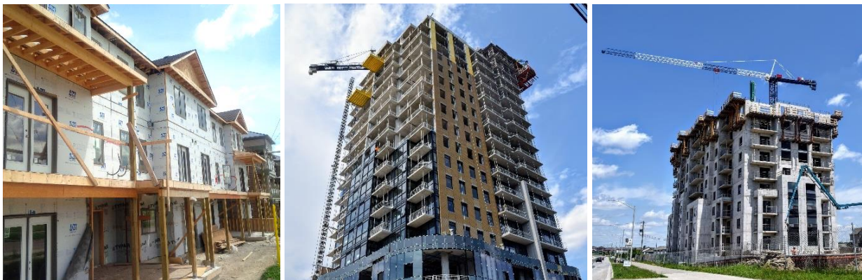
Figure 72 - New Housing Under Construction
