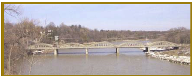
The Bridgeport Bridge was rebuilt as public works project during the Great Depression and contributes to Village character.
