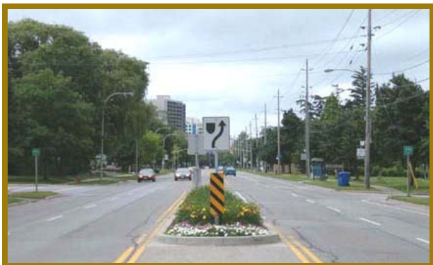
Landscaped pedestrian refuge islands improve pedestrian access across major corridors and contribute to the streetscape.
