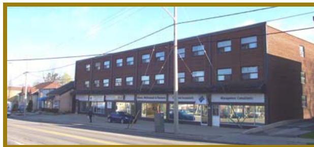
Streetscape clutter is eliminated when signs are fully integrated into the building design and relate to individual store fronts.
