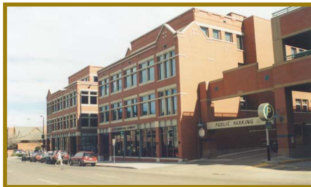
Public parking structures with grade related uses improve streetscape appearance and function.
