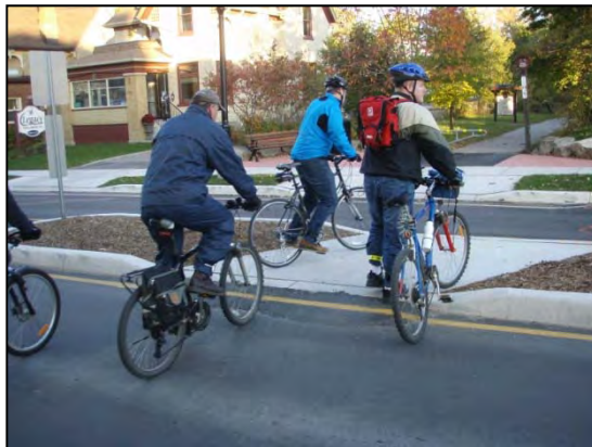
Iron Horse Trail crossing at Queen Street—new median refuge allows crossing one direction of traffic at a time with enough room on median to wait with a bicycle
