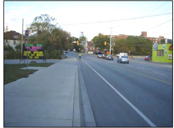
Looking east on Victoria Road at the westbound bike lane
