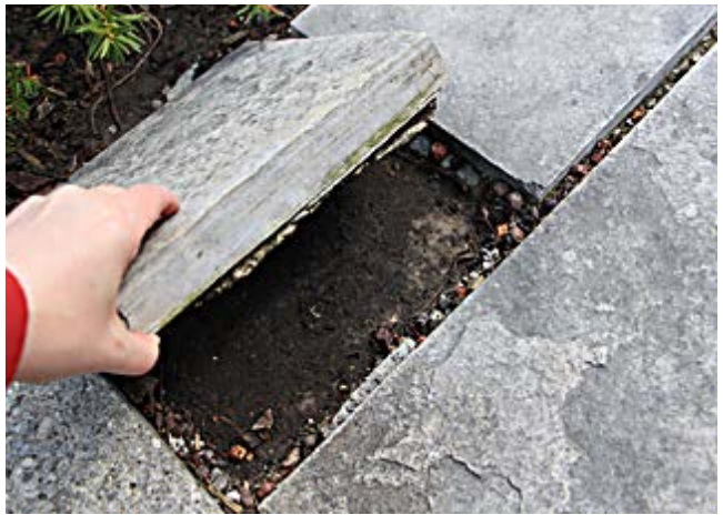
Fig. 33 Existing pavers within the north public gardens are set on a sand base.
