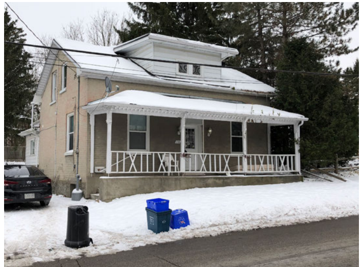
House on Pinnacle Drive (Photo: Carl Bray, Bray Heritage)
