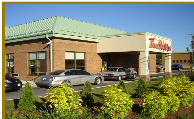
Portico provided for weather protection at drive-through window.
