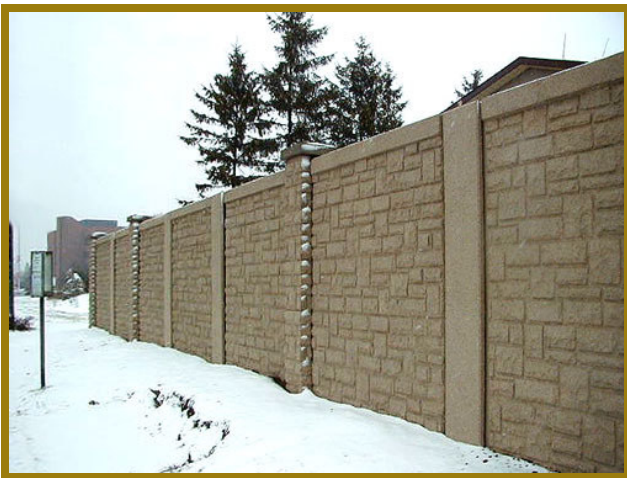
An example of a wall used as an acoustic barrier.
