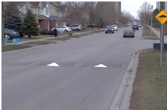
Speed Humps/Cushions or Raised Crosswalks
