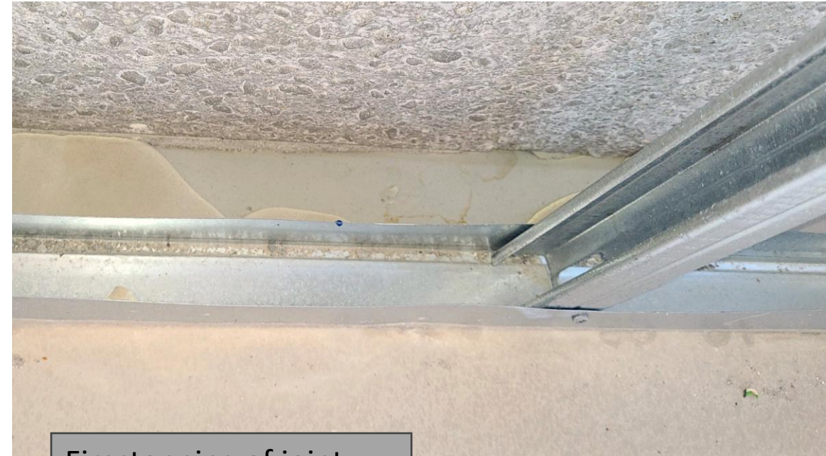
Firestopping of joint where floor abuts wall
