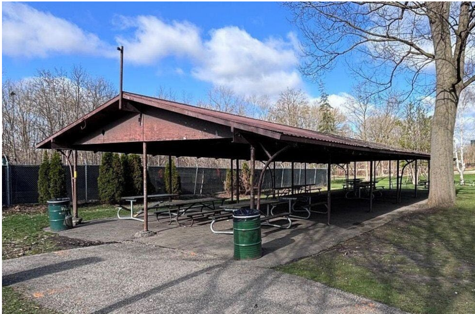
Figure 3: Existing picnic shelter
