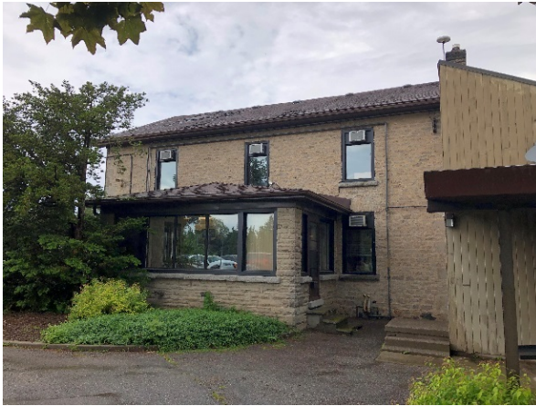
Plate 21: Clubhouse, looking northwest
