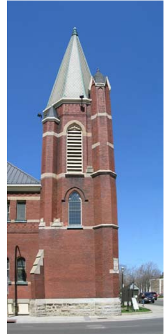
St. Andrews Church – slate, brick and stone landmark
