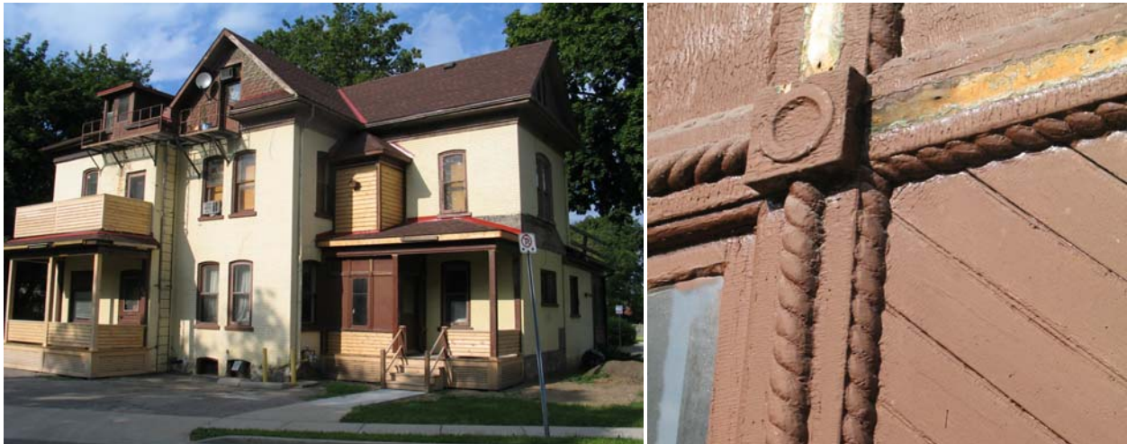
115 Lancaster Street East - repair of wood trim
