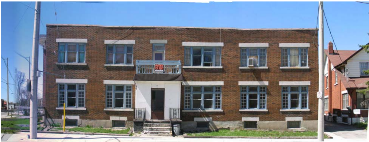
58-60 Weber Street, 96 Young Street, two faced addition
