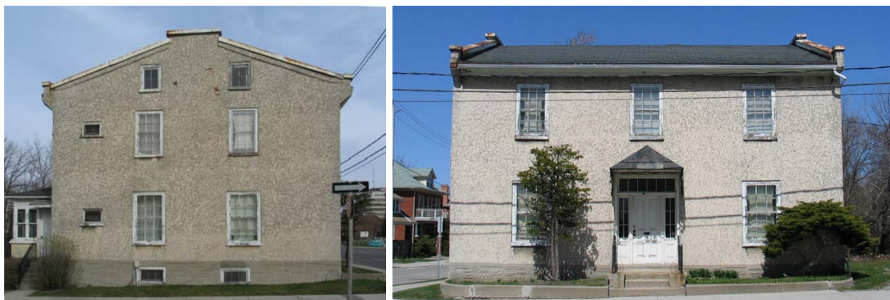
74 Weber Street West and side elevation
