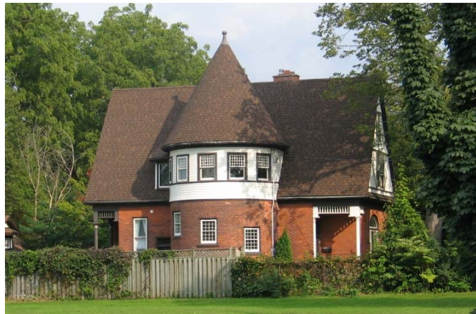
Example of appropriate, well-maintained roofing material, and colour for heritage buildings
