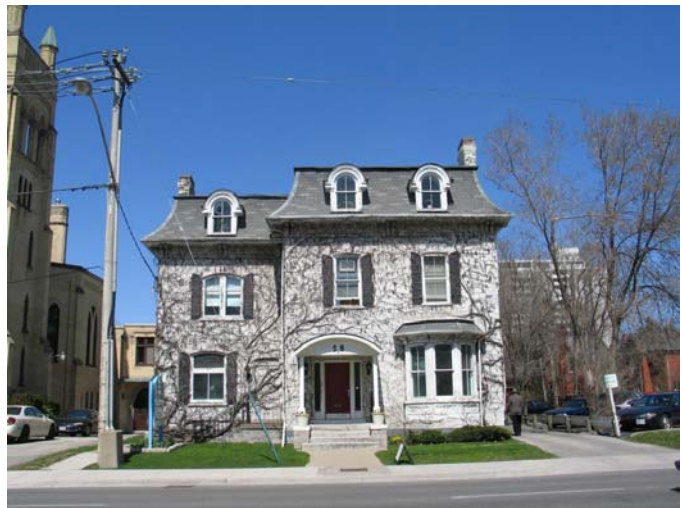
28 Weber Street West – Second Empire style with mansard roof and dormer windows
