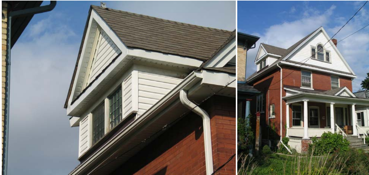
34 Ellen Street East -Dormer reclad
