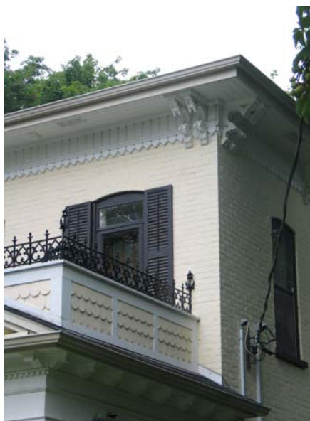
124 Young Street – ventilated soffit
