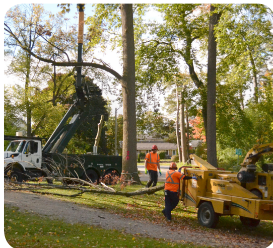
Large tree removal requires skilled tree workers and specialized equipment.
