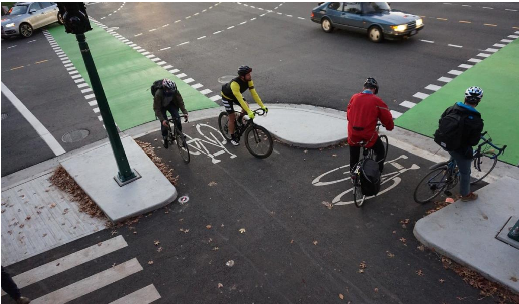
A separated intersection in Vancouver. 60
