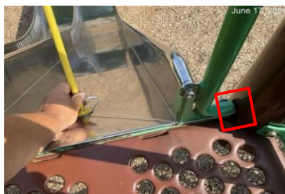
#17 - Area 2 - String entanglement hazard present on the right side of the double stainless steel slide (between barrier rail and support post)
