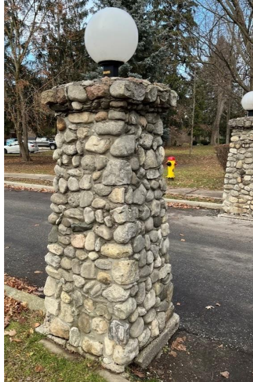
Figure 43: Entry Feature at Schneider Avenue
