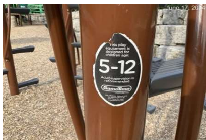
#22 - Manufacturer's labels are present in Areas 1, 2 & 3
