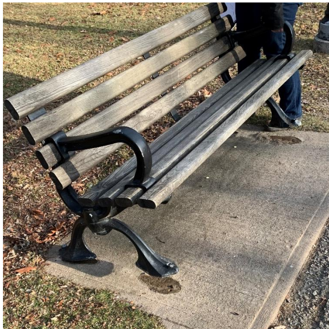
Figure 11: Memorial Bench Missing Mounting Bolts
