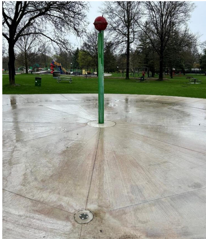
Figure 2: Existing Above Ground Splashpad Infrastructure Consisting of Misting Nozzles and Jet Nozzles Spraying Horizontally, called a Melvinator
