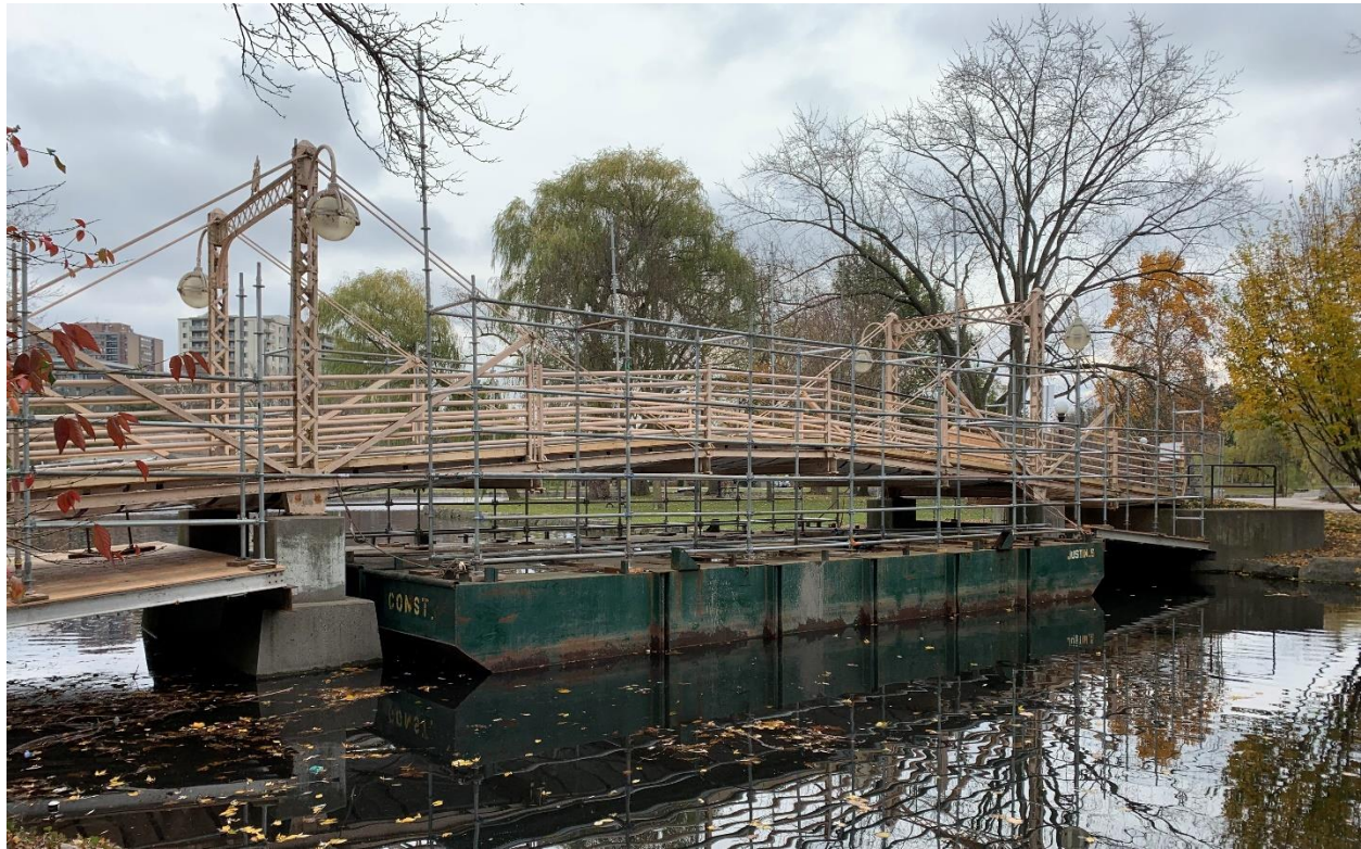
Figure 77: Pedestrian Bridge 877 – November 2024 Construction
