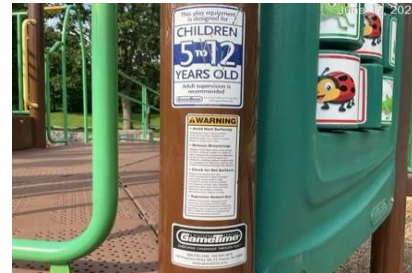
#21 - Manufacturer's labels are present in Areas 1, 2 & 3
