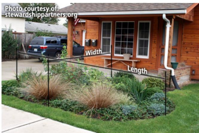
After entering the length and width of the rain garden into the form you must also enter the depth of the bioretention media beneath the rain garden and to enter the depth of the gravel layer located beneath the bioretention media. Typically, the bioretention media ranges in depth from 0.35m to 1m and the gravel layer, if present, is typically about 0.3m deep. If you do not know the depth dimensions enter 0.35 meters depth for bioretention media and 0.0 meters depth for the gravel layer.
