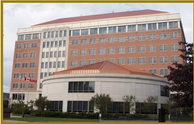
Figure 7.6: The sloped roof of this civic building fully screens rooftop mechanical equipment and creates an attractive roofline.
