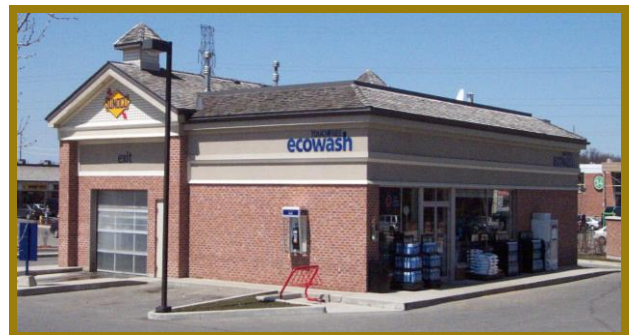
Figure 7.9: The articulated roofline on this gas station and car wash fully screens rooftop mechanical equipment and helps create an attractive building design.
