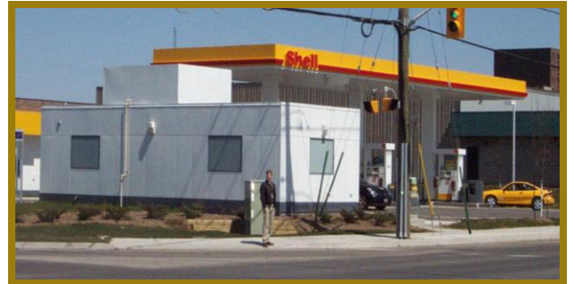
Figure 7.8: Although the rooftop equipment on this gas station is fully screened with materials matching the building, the enclosure is not well-integrated with the building form.
