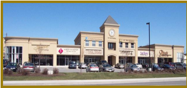
Figure 7.3: Rooftop equipment screening methods used on this building include parapets, an articulated roofline, and centralized location of equipment.
