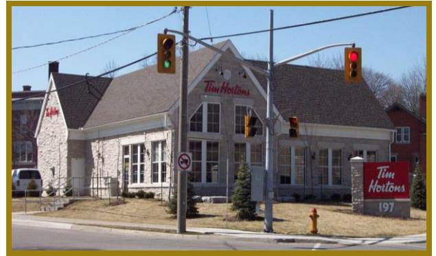
Figure 7.5: The peaked roof of this low-rise building screens all rooftop equipment and helps define the intersection where the building is situated.
