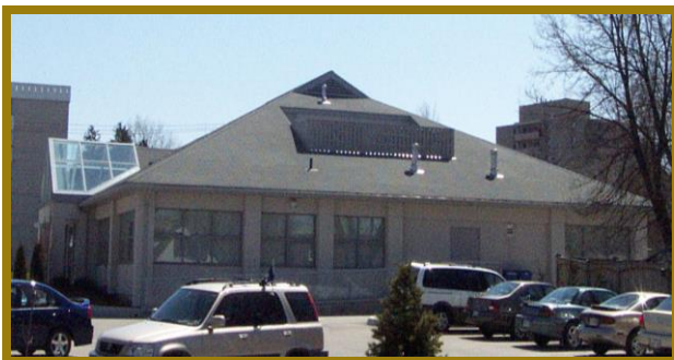
Figure 7.4: Rooftop mechanical equipment for this building is hidden by a screening wall that is integrated with the building design. The screening also articulates the roof elevation.
